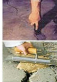
shatter; excellent for anchoring machinery and vibrating equipment as well as cracks.
